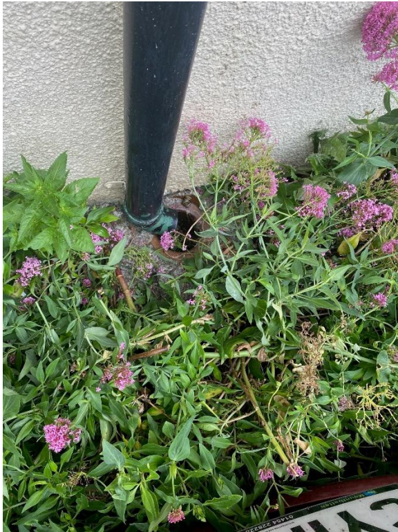
Photo 3 – Rainwater Downpipe and gully on side elevation
