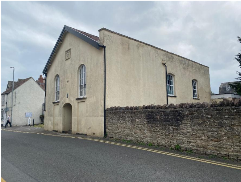
Photo 2 – Chapel Road elevation and entry point for National Grid Cable
